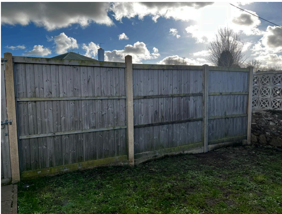
(An Image of the repaired fence)
